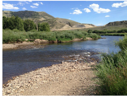
Figure 1 Engineered Riffle Grade Control Structure provides reliable irrigation diversions and critical aquatic habitat.
