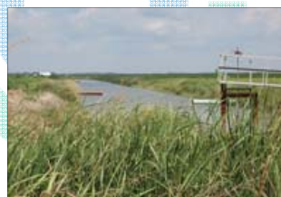
Drop pipes used to discharge runoff into waterbody to avoid erosion
