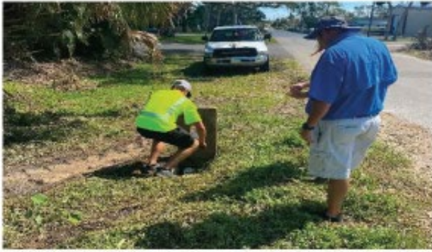
Checking for Leaks
