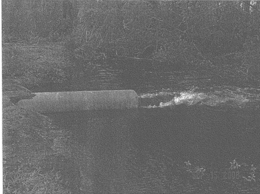
Pumps working to Drain Fields of Water
