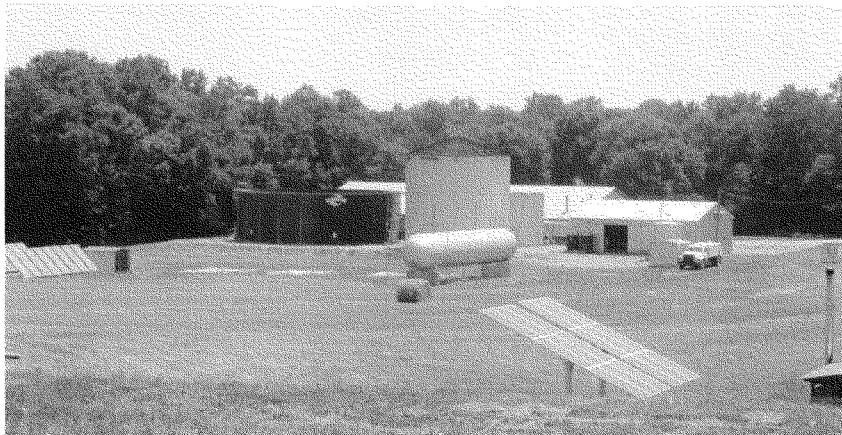
Figure 5. On-Farm Poultry-Litter Anaerobic Digester in Mississippi Integrated with Solar Energy
