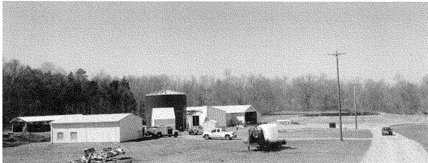
Figure 6. A New On-Farm Poultry-Litter Anaerobic Digester in Kentucky
